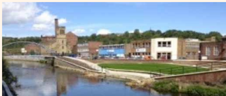
River flood risk management scheme in Sheffield (UK). This retrofit bank raising has been landscaped to promote recreational use and improve visual appearance and can be classed as WSUD.
